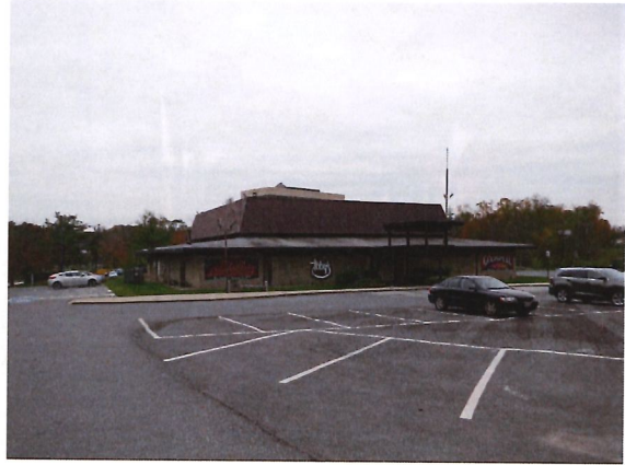
Typical view of improvements on subject property, looking southeasterly
