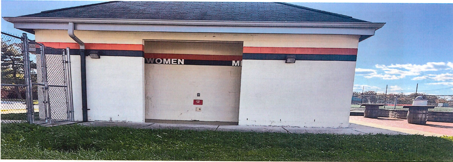
OMHS indoor stadium bathrooms since 2011
