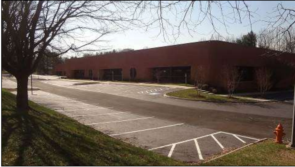
Subject building & parking lot looking southeast
