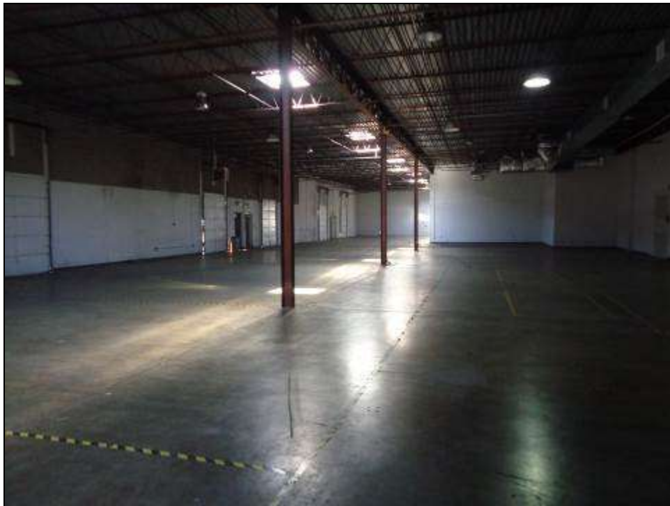
Warehouse area at rear of Suite E in southern corner
