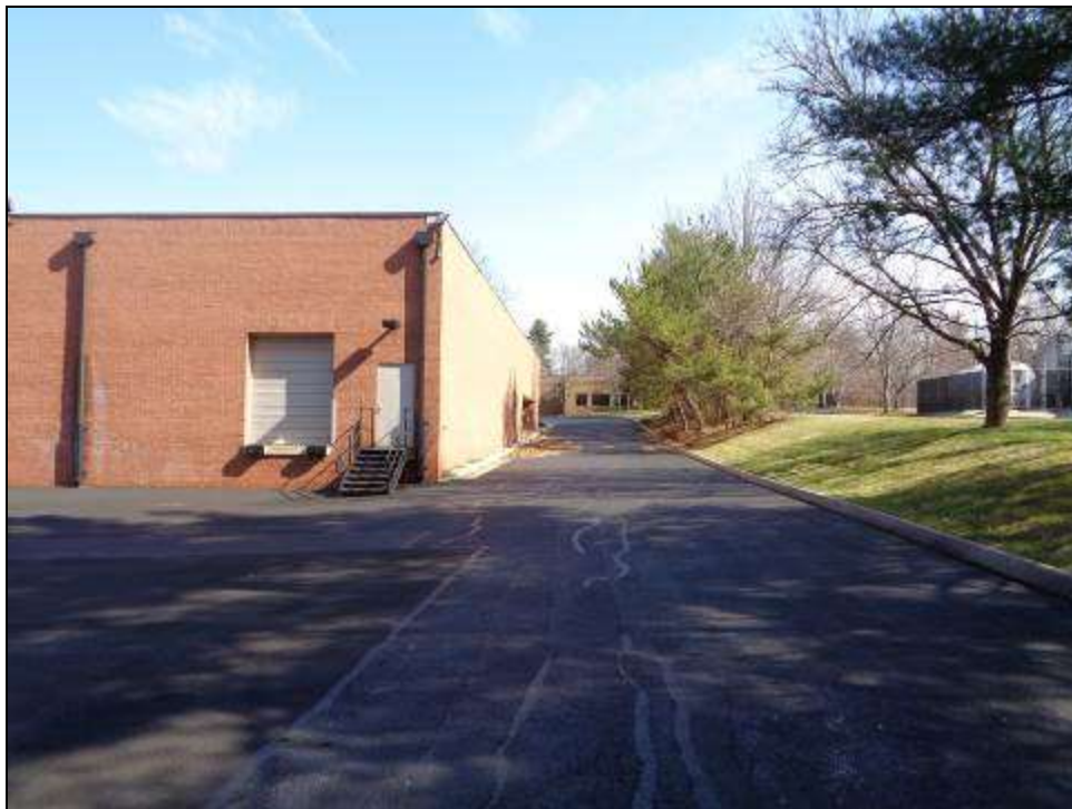
Southeast subject side looking toward Mendenhall Court
