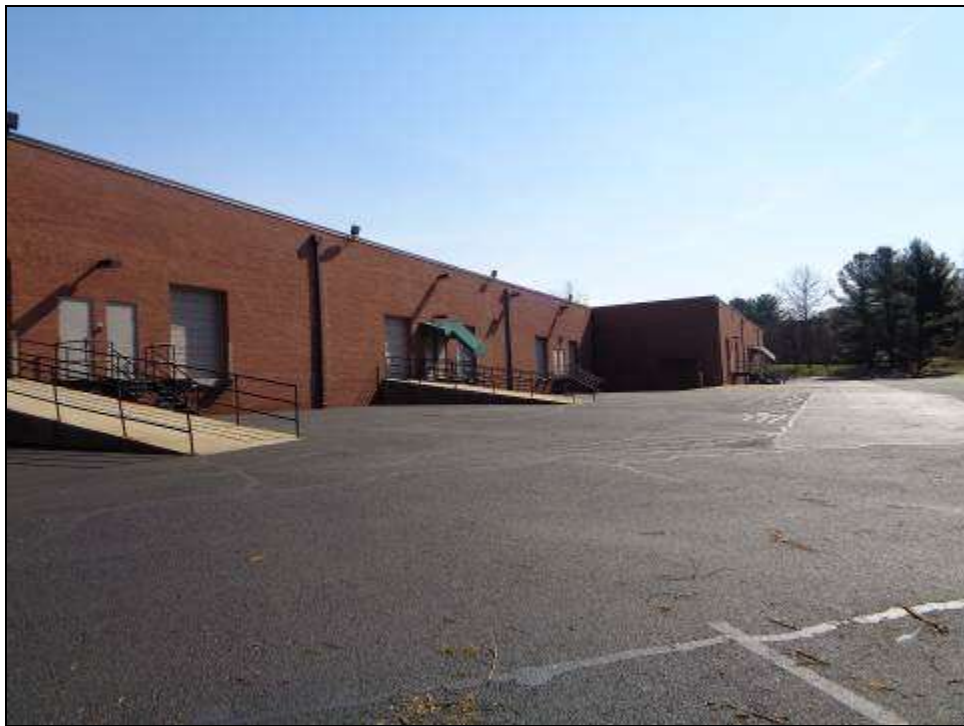
Subject rear looking east
