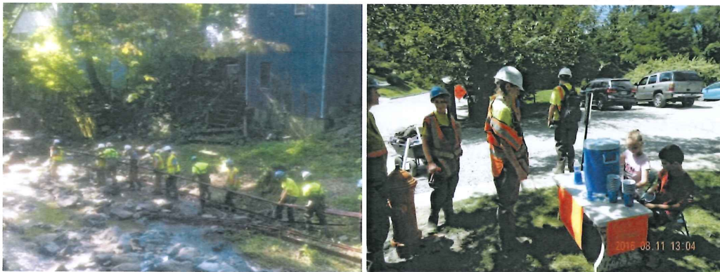
READY crew conducting post flood clean-up in Ellicott City.
