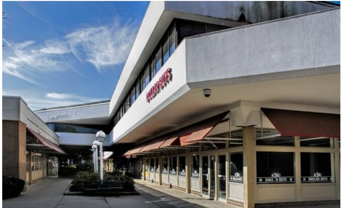
Existing building at the LRVC
