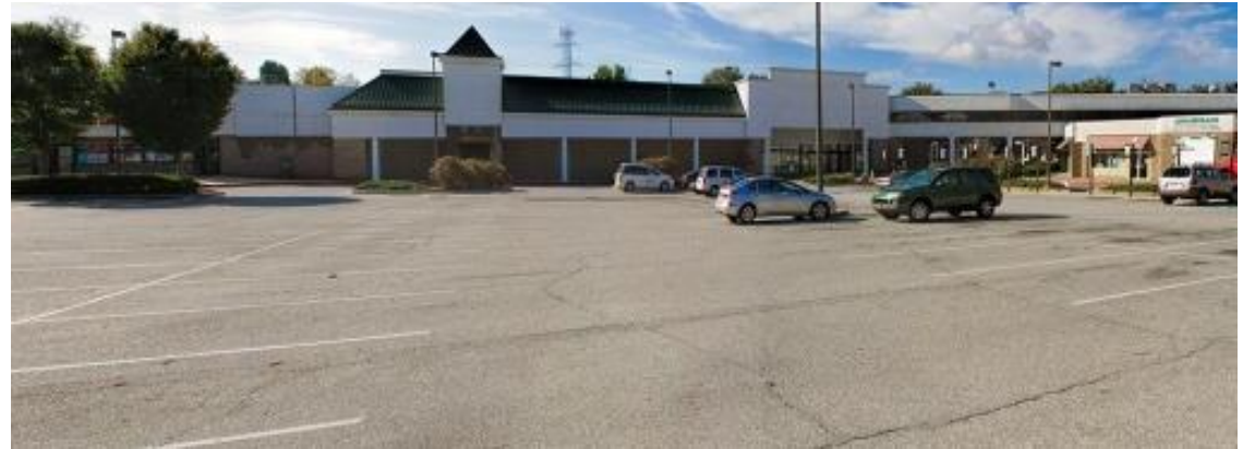
Parking lot in front of the vacant grocery space
