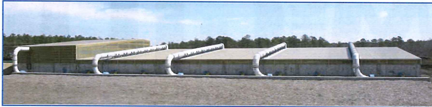
McGill-Waverly is the largest enclosed composting facility in Virginia. In the foreground is the biofilter, designed to remove odors and particulates from process air.
