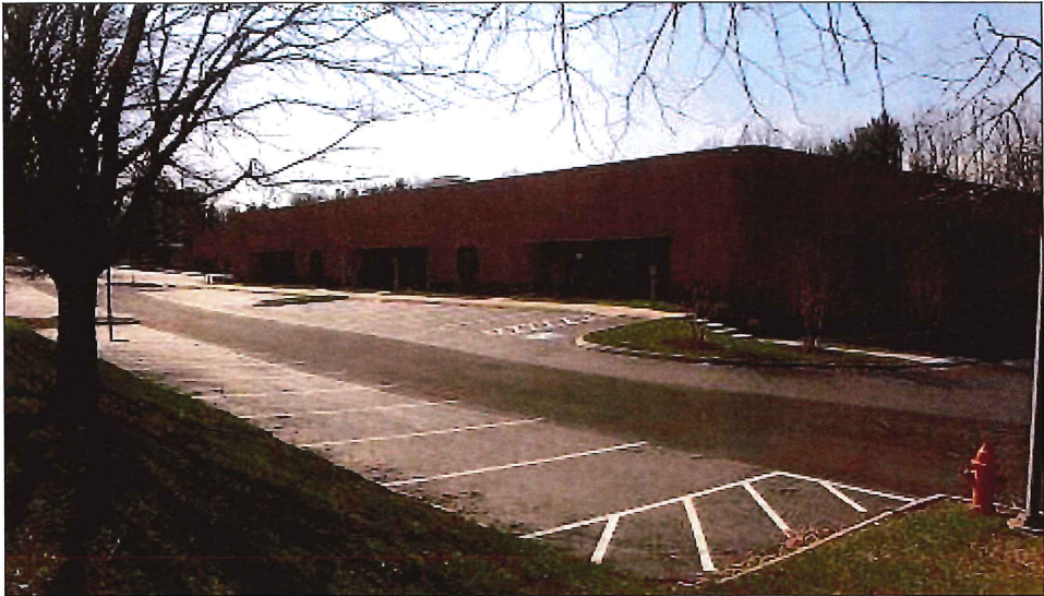
Subject building & parking lot looking southeast
