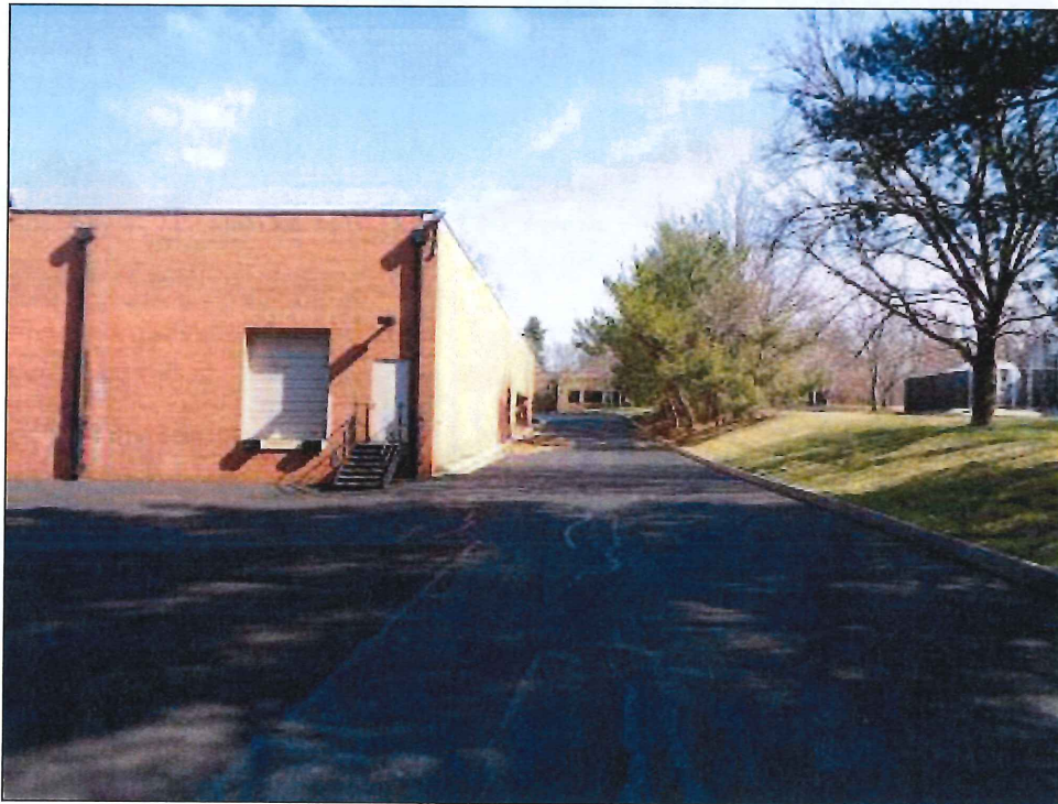
Southeast subject side looking toward Mendenhall Court
