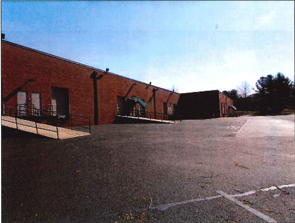
Subject rear looking east
