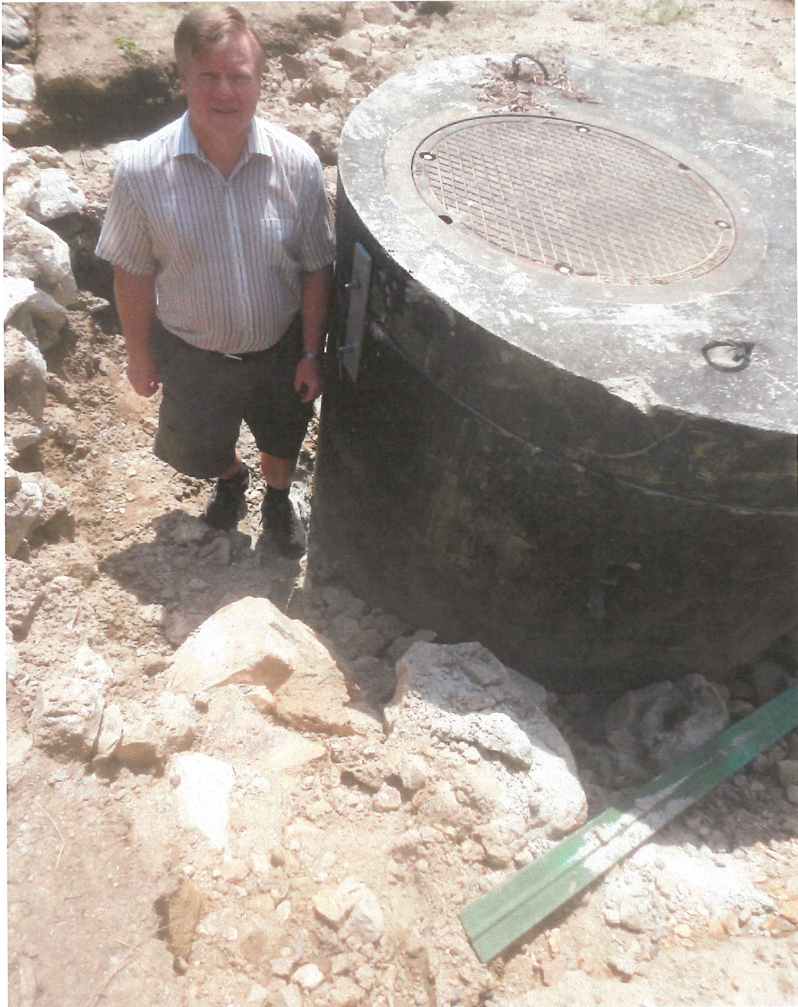
Sewer manhole near proposed path August 2016
