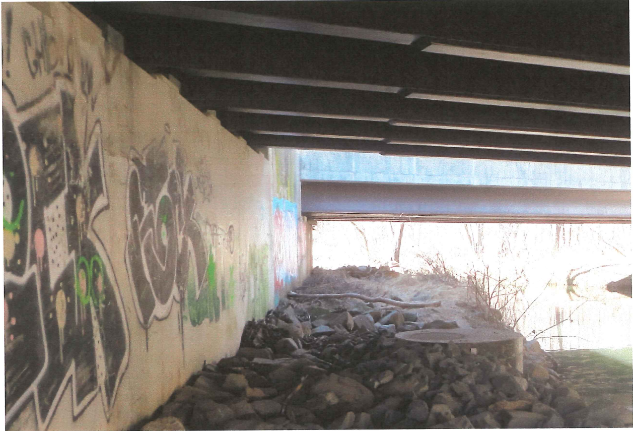
Sewer Manhole under Route 29 bridge February 2017
