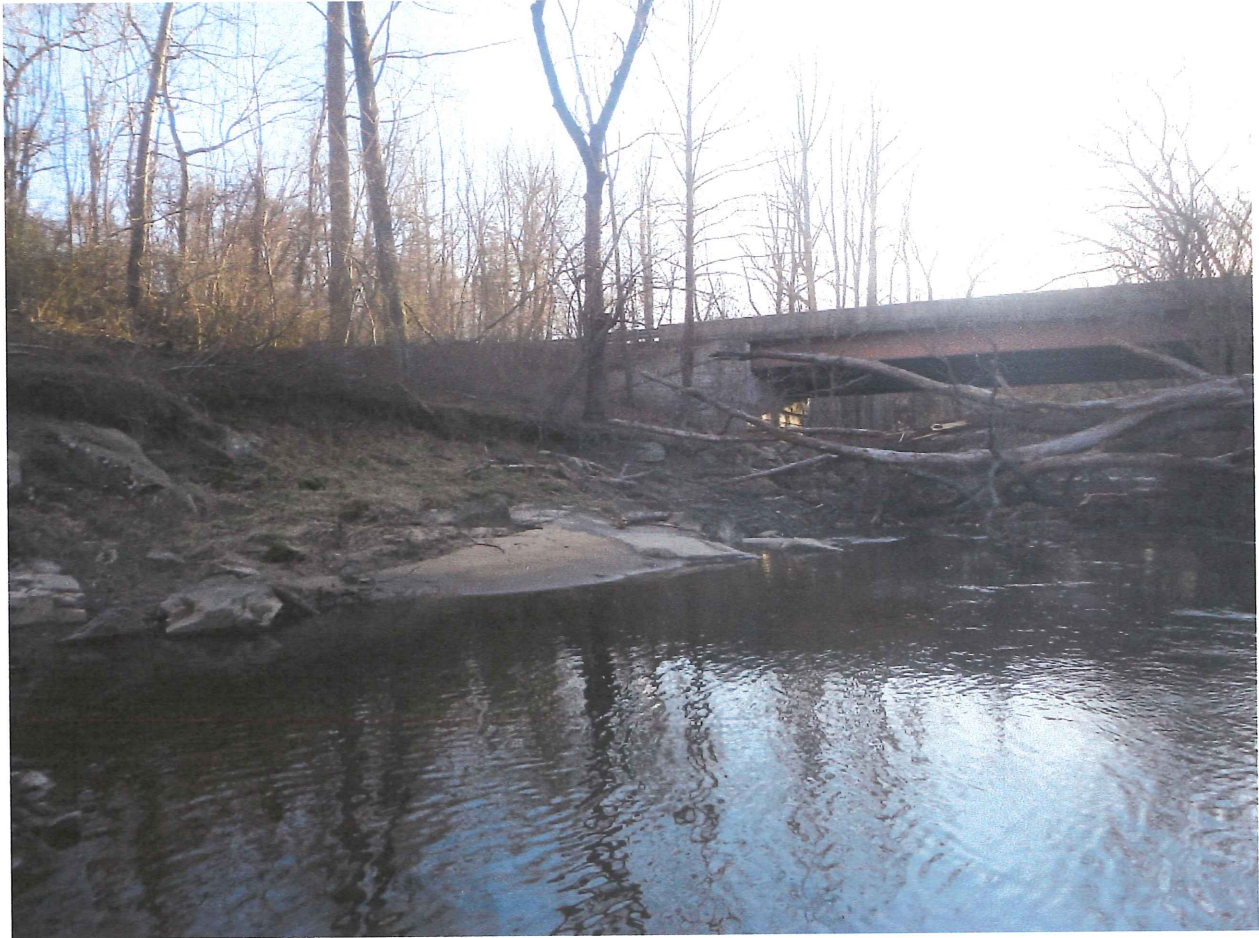
Tree blocking river at Stevens Forrest Road Bridge Feb. 2018
