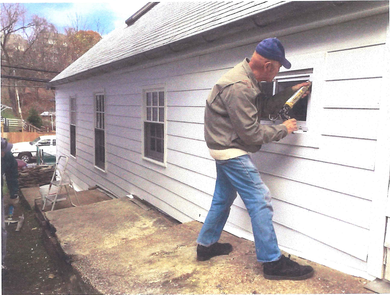
Exterior flood victim home after new siding, roof and windows.
