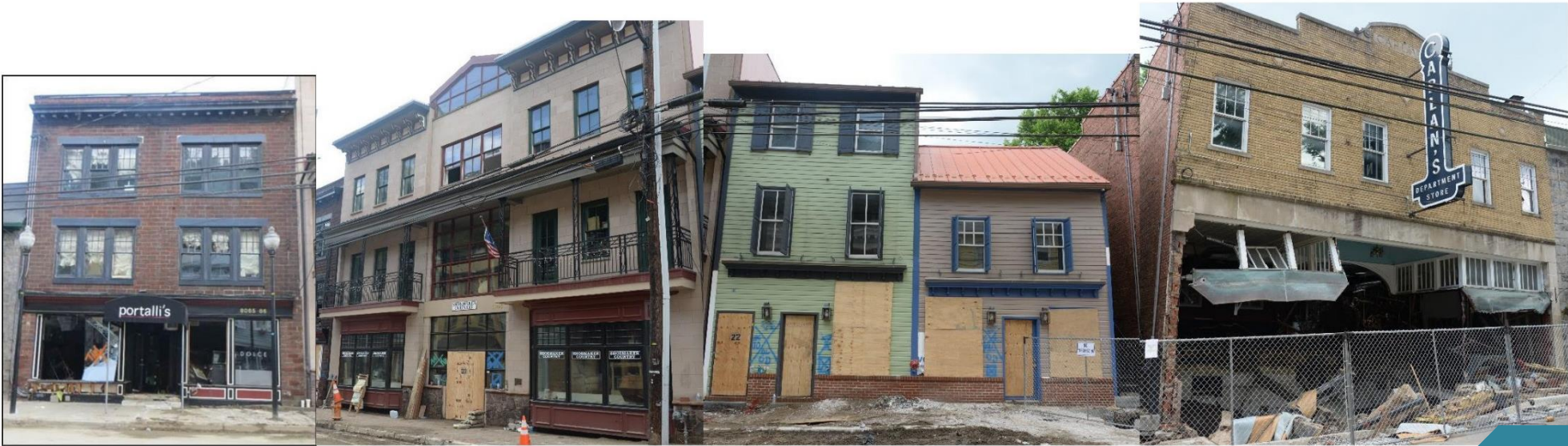
Portalli's 8085 Main St. Brick: c. 1920s, c. 2000
