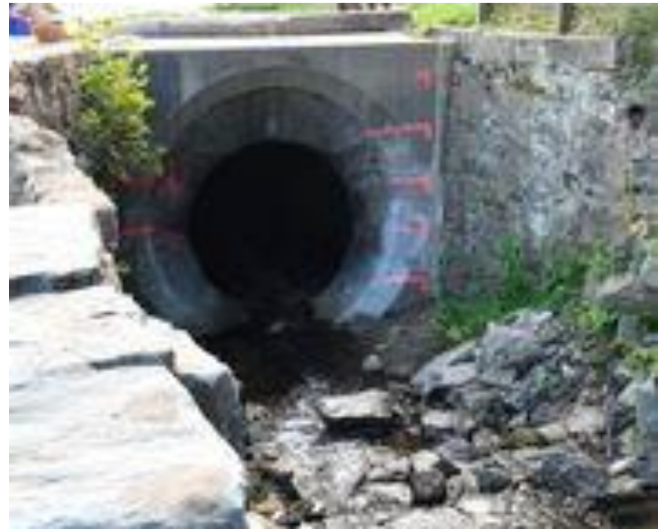
8600 Main St. Culvert; 84 inch diameter
