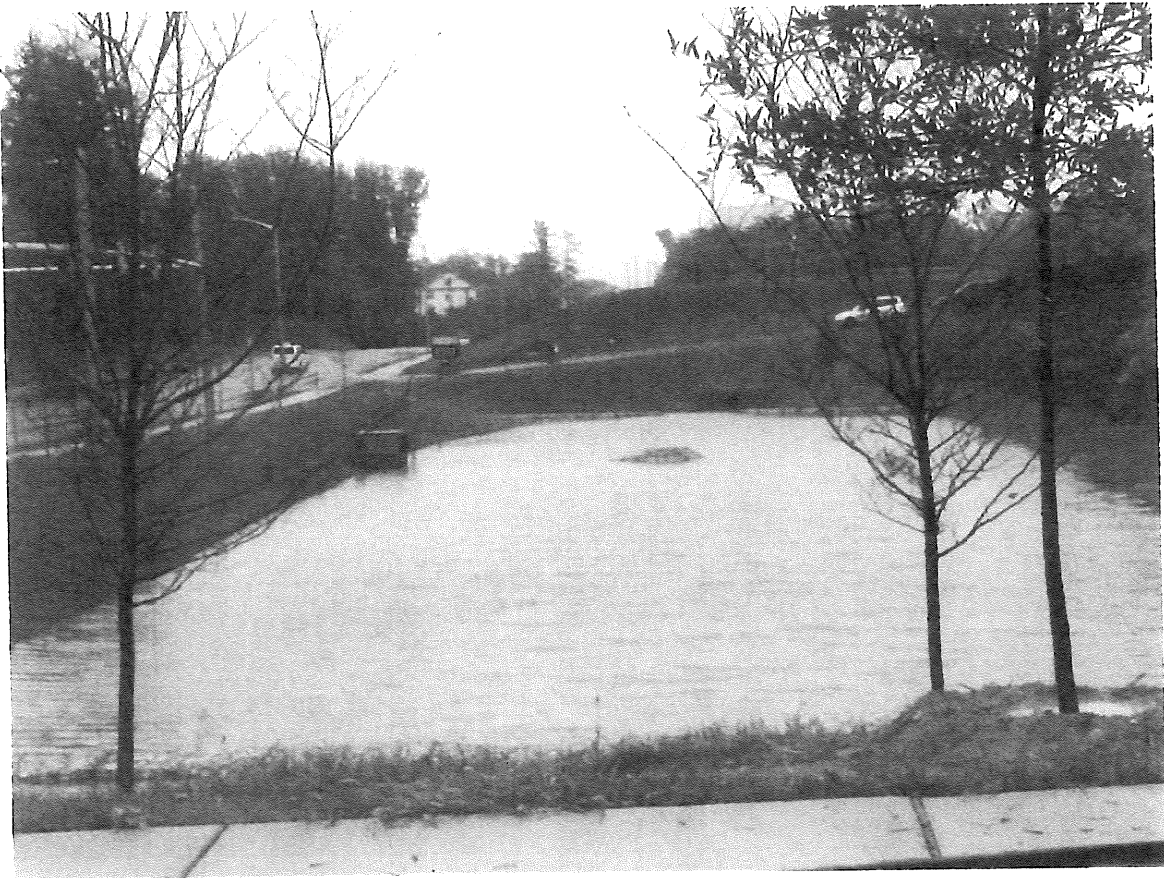
This shows the dry SWM on Lyons Mill road working during a very rainy day
