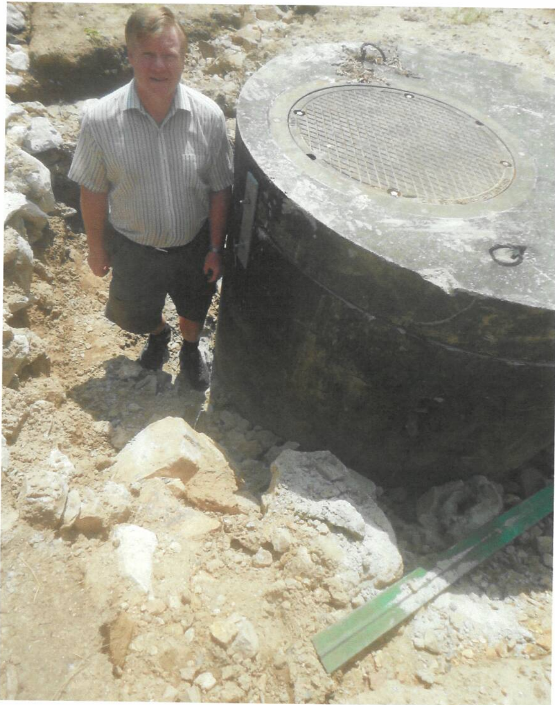
Sewer manhole near proposed path August 2016
