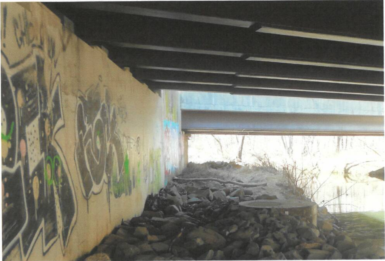
Sewer Manhole under Route 29 bridge February 2017
