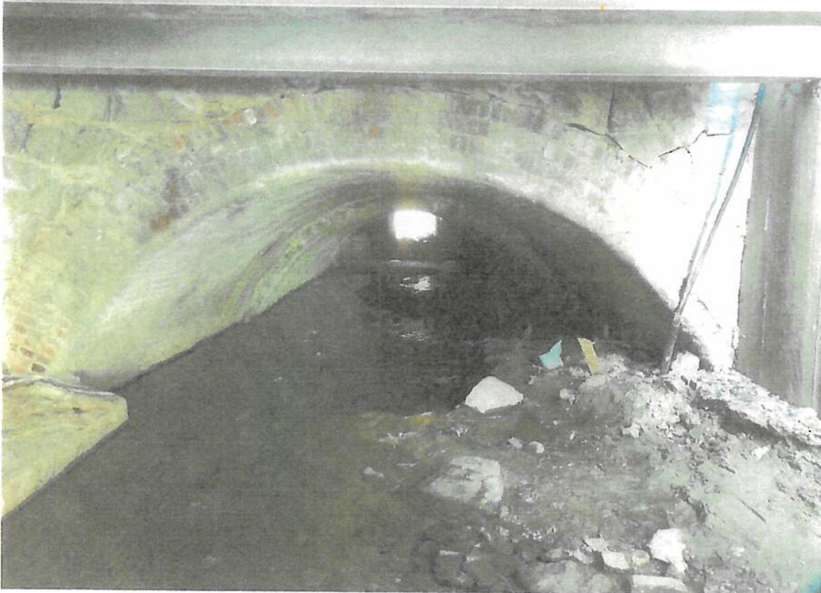
This is the channel and Arched culvert under main street. The culvert restricts the volume of water flowing thru the Hudson channel , it clogs
