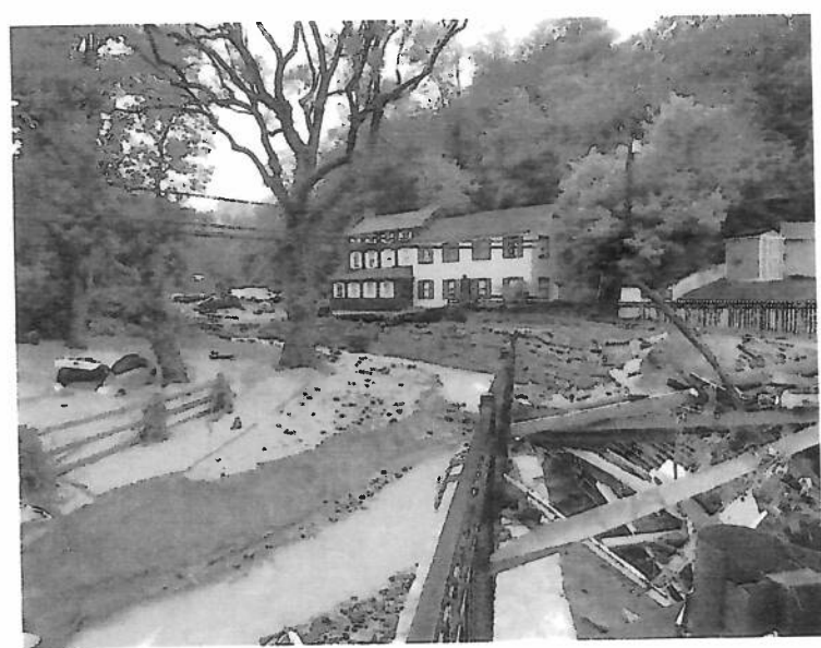
2018 Flood damage at Court Ave shows sediment and debris from Ellicott Mills wash out
