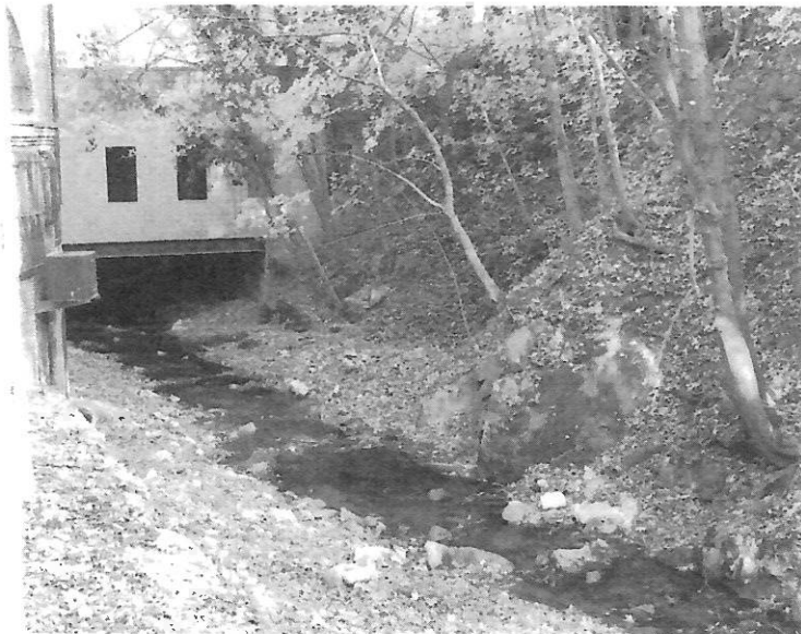
Ceplan's before 2018 Flood during reconstruction.
