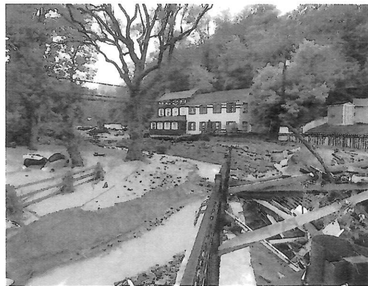
2018 Flood damage at Court Ave shows sediment and debris from Ellicott Mills wash out
