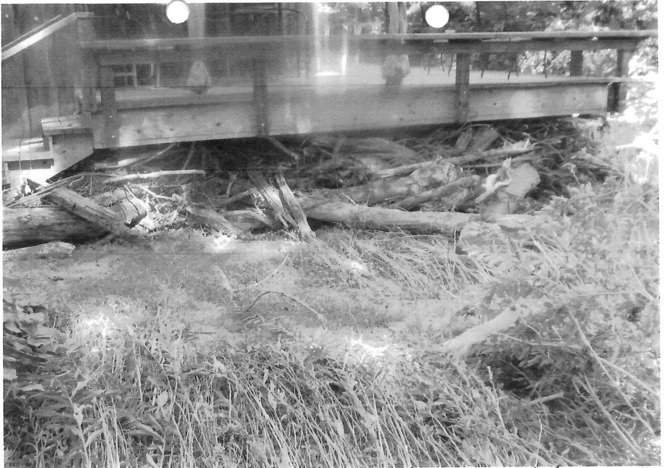
Merryman Street 2016 Flood, Porch has collapsed in 2018 Flood
