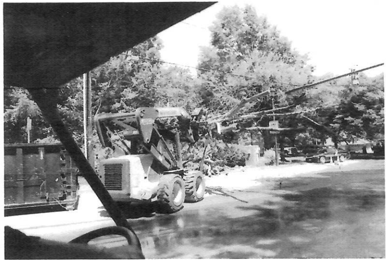
2016 debris clean up at Ellizott Mills
