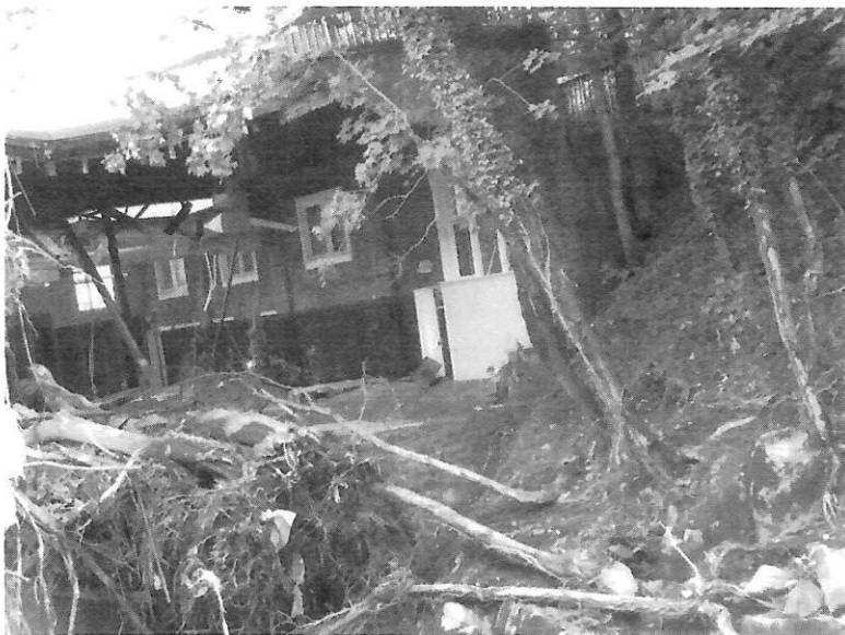
Ceplan's after 2018 Flood, shows how much floating debris came thru the building
