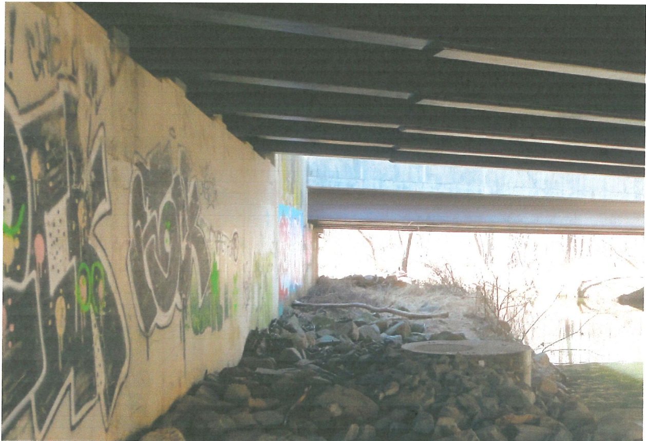
Sewer Manhole under Route 29 bridge February 2017
