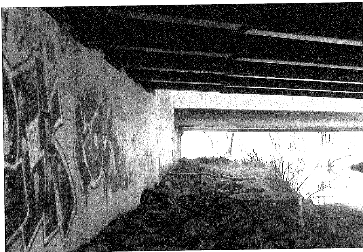
Sewer Manhole under Route 29 bridge February 2017
