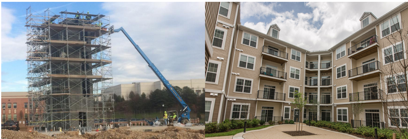
Oxford Square construction.
