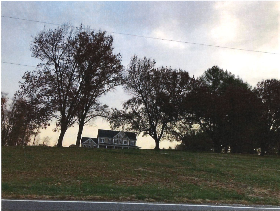
New house built on the knoll in the background along Old Frederick Road.
