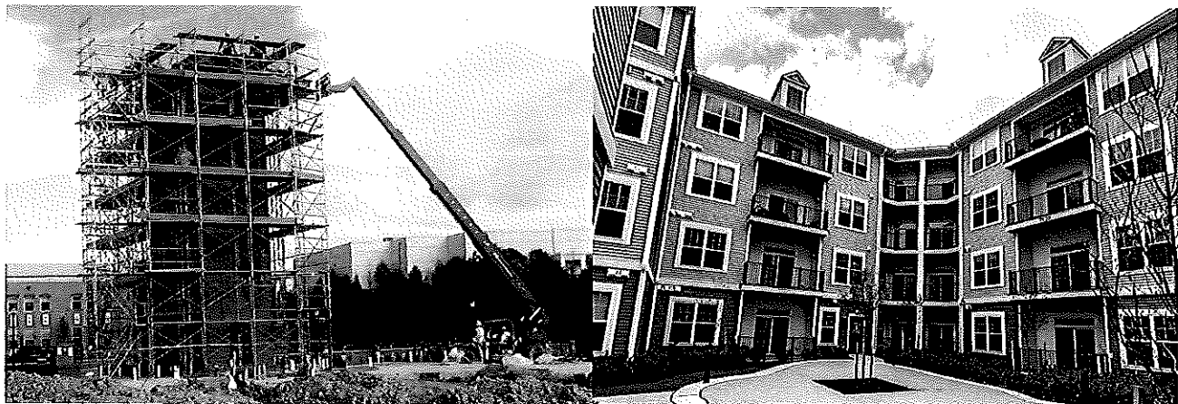
Oxford Square construction.
