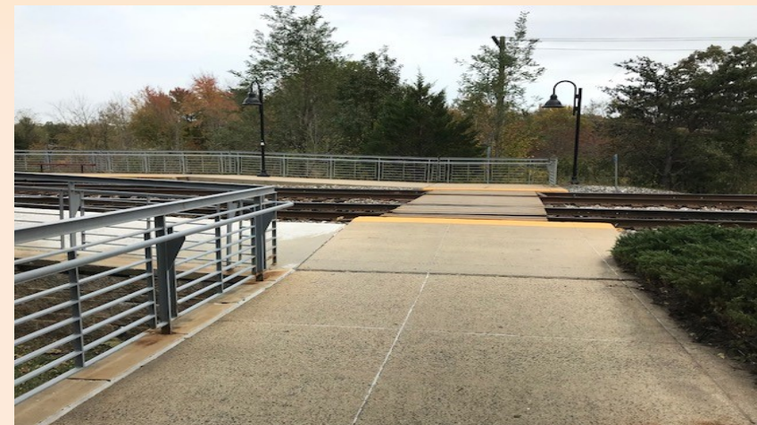
Figure 11: Dorsey MARC Station at-grade crossing to the northbound platform
