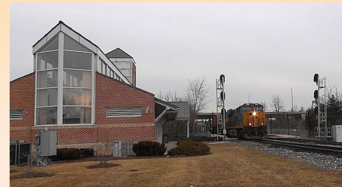
Figure 4: Northview - Station southbound platform
