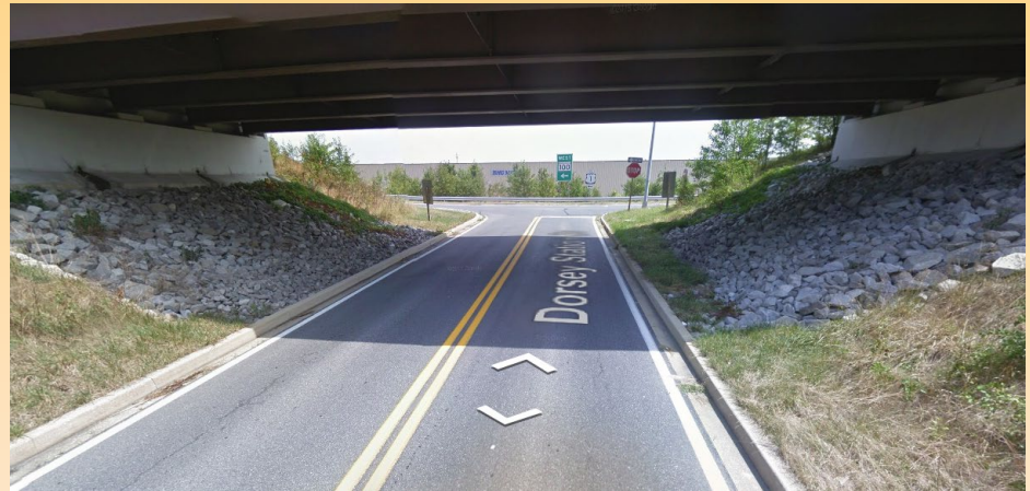
Figure 13: Dorsey Station Drive under MD US 100 – view from Station towards MD US 100 Exit 7 ramps
