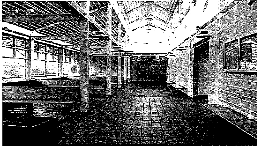
Figure 10: Dorsey MARC Station lobby
