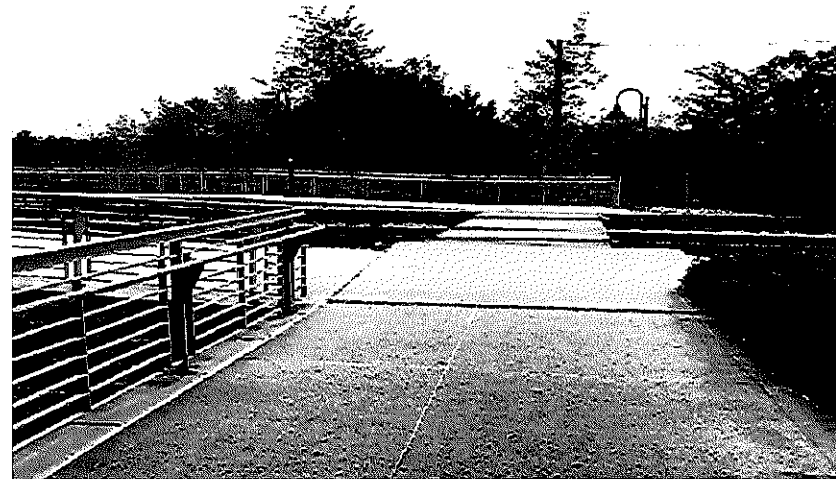
Figure 11: Dorsey MARC Station at-grade crossing to the northbound platform
