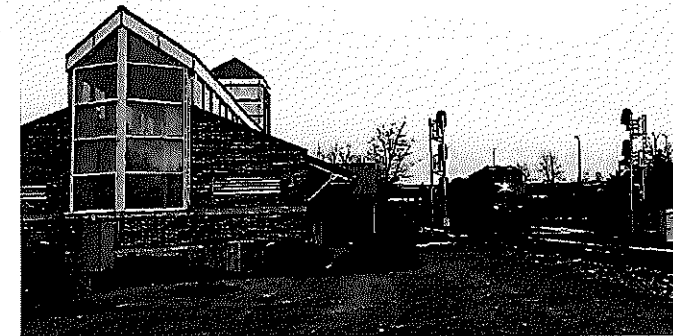
Figure 4: Northview - Station southbound platform
