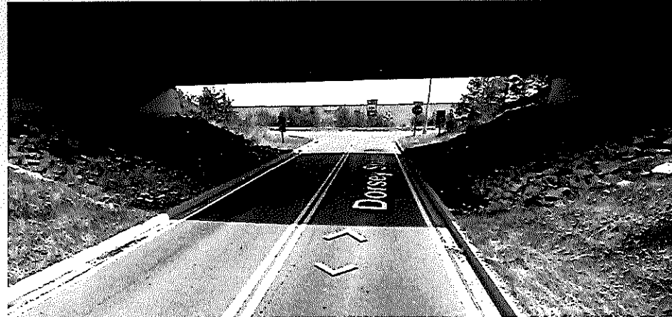
Figure 13: Dorsey Station Drive under MD US 100 – view from Station towards MD US 100 Exit 7 ramps
