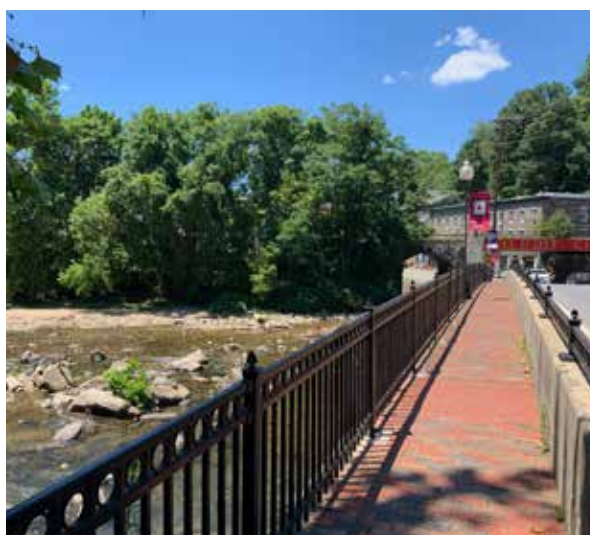
Figure 129: Opportunity to Enhance the Gateway Experience by Opening Views to the B&O Museum from the Patapsco River Bridge
