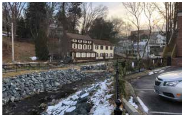
Figure 47: Daylighted Section of the Hudson Branch in Lot F After the Reconstruction Following the 2018 Flood
