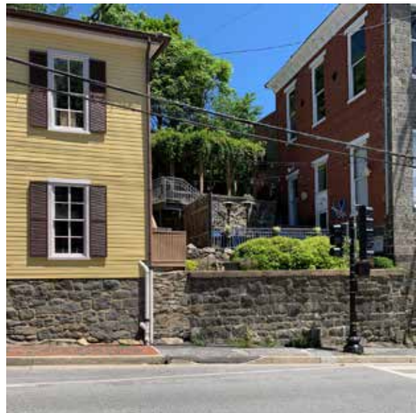
Figure 20: Typical Materials of Mid-19th Century Buildings in Ellicott City Include Stone, Brick and Wood Frame
