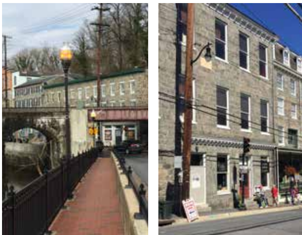
Figure 101: Existing Ornamental Lighting
