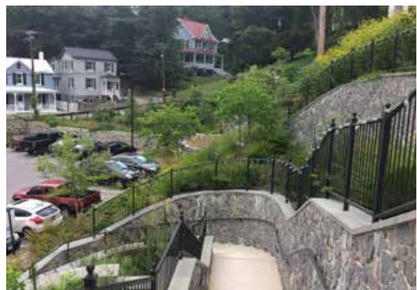
Figure 208: The Lot E Staircase Creates a Memorable Link Between the Courthouse Area and Main Street
