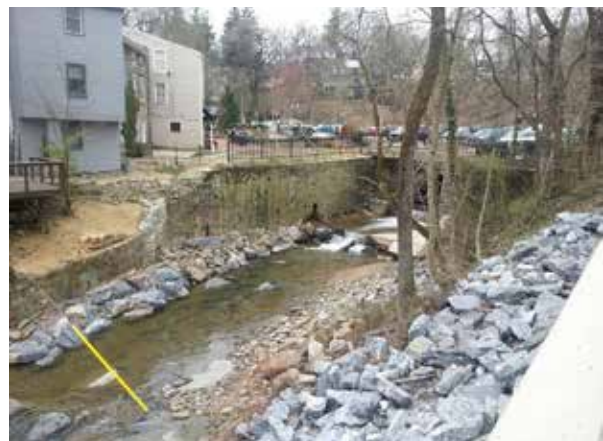
Figure 154: Hudson Branch along Tonge Row and Hamilton Street
