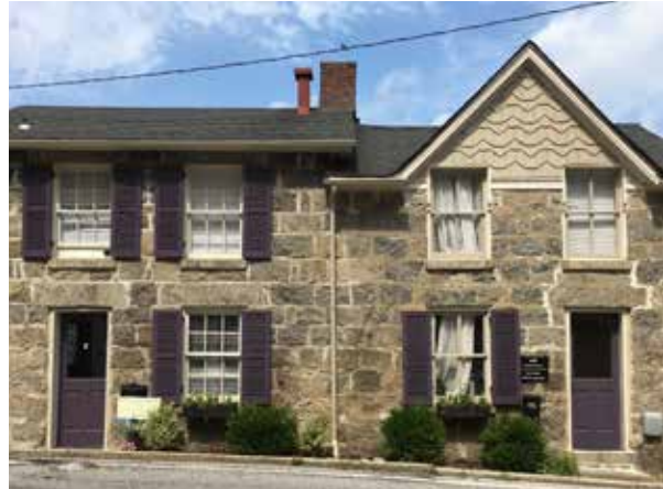
Figure 27: Rehabilitated Tonge Row Facades as part of Howard County Facade Improvement Program
