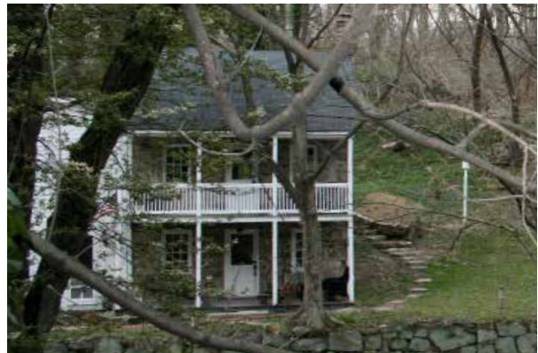
Figure 16: Historic West Main Street House Overlooking Former Mill Race
