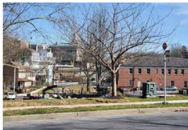
Figure 176: Lot F and Potential North Tunnel Entrance Area after 2019 Reconstruction
