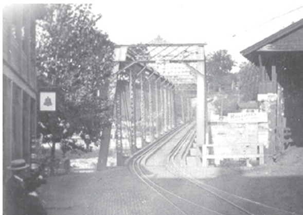
Figure 118: Historic Photo of Trolley #9 Bridge, Credit: Baltimore County Public Library/MD Covered Bridges
