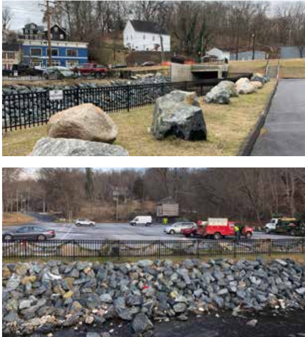
Figure 71: Boulders and Fencing Were Placed Between Lot F and the Stream Channel as Part of the Parking Lot's 2019 Reconfiguration.
