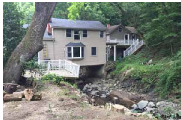
Figure 198: Existing House Spanning the Hudson Branch Channel in the West End
