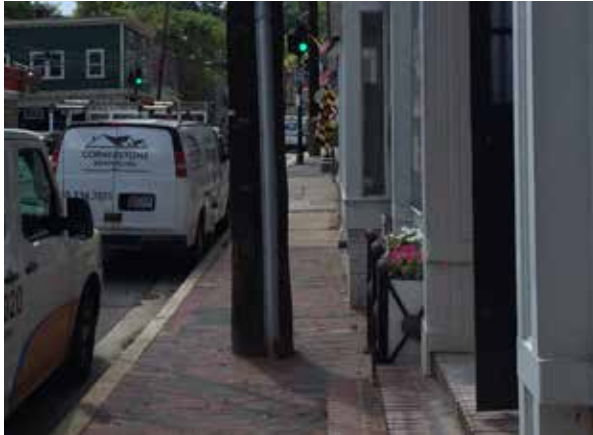
Figure 66: Utility Poles Often Limit Usable Sidewalk Space
