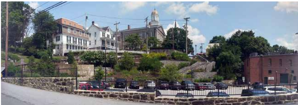
Figure 155: The Lot E Staircase Strengthens the Connection Between the Courthouse and Main St
