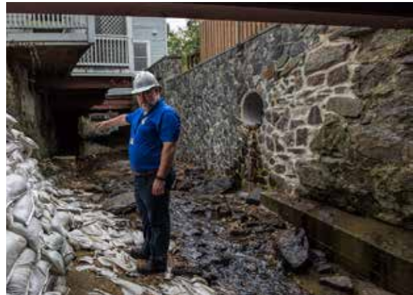
Figure 143: Character of Existing Stone Channel Walls
