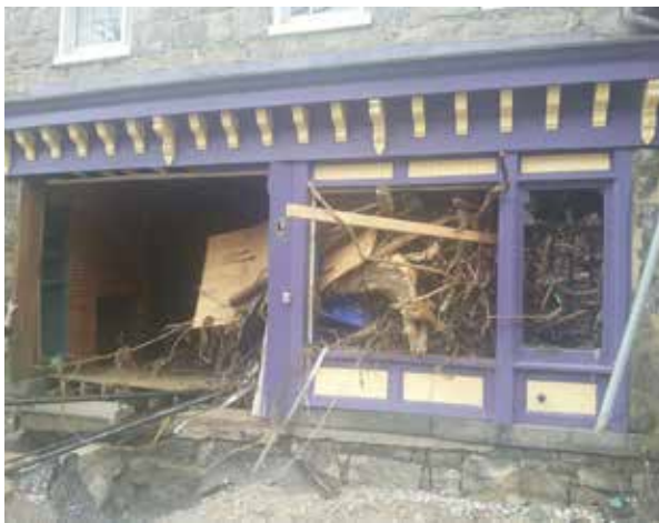
Figure 38: Vulnerable Tree Cover Along Stream Edges Creates the Potential for Debris Mobilization and Damage Downstream (Top); Tree Lodged in Building (Bottom)
