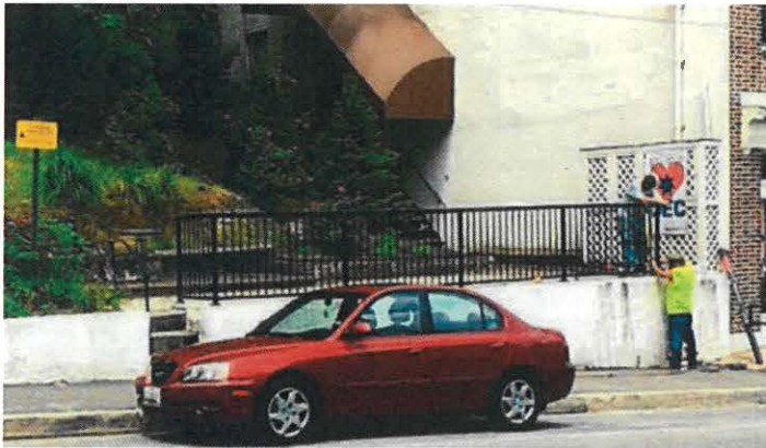
Figure 22 - Fence installed and approved in July 2020.
