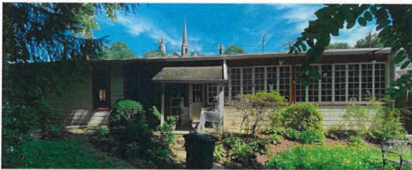
Figure 17 - Existing rear view
