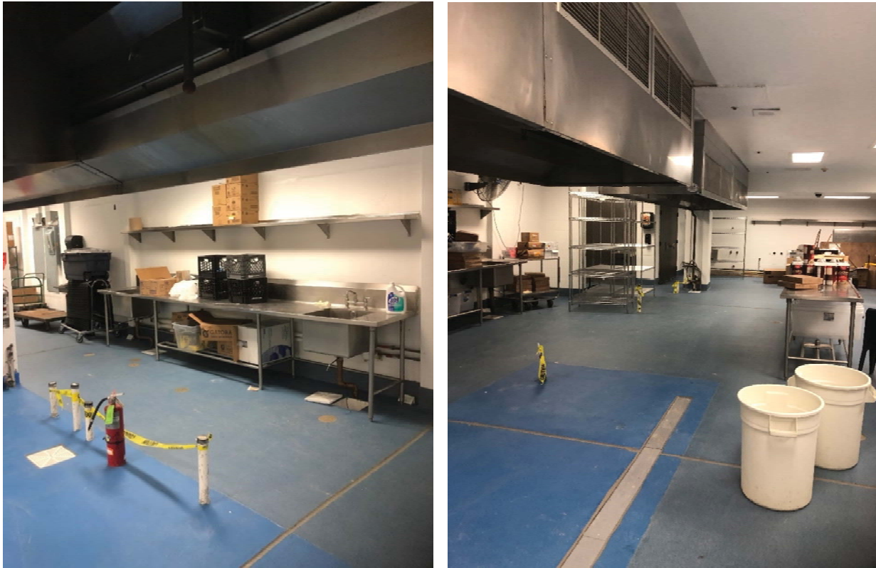
Figure 3. HCDC's kitchen undergoing renovation as observed by DHS OIG on December 17, 2019.
