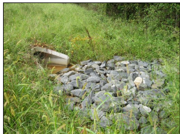
12. View of stormwater outlet located at the north end of the subject site
