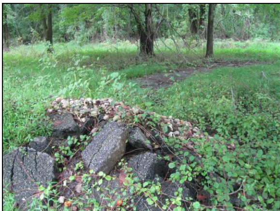
8. View of broken asphalt and walkway at the north/central area of the subject site
