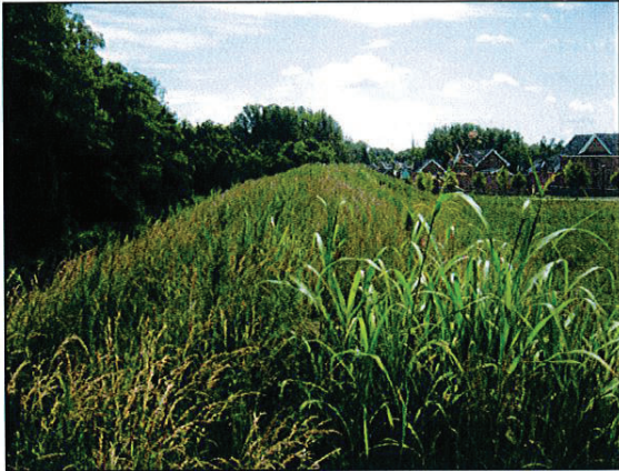
1. View of berm cap facing east
