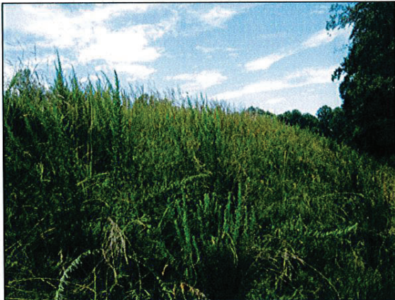
2. View of north side of berm cap facing west
