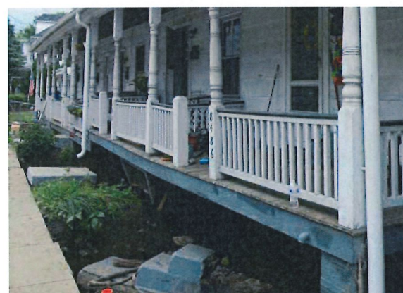
Figure 201: Foundations Scoured by Floodwaters in the West End
