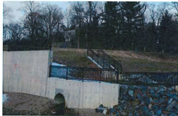
Figure 46: Existing Culverted Stream Outfall in Lot F After the Reconstruction Following the 2018 Flood
