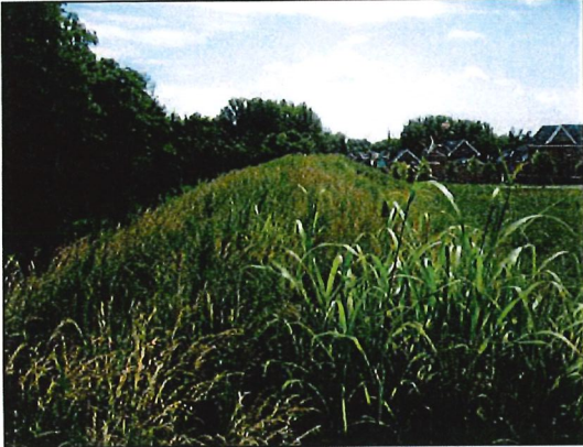
1. View of berm cap facing east
