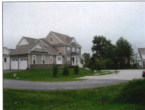
5. View of adjacent residence located to the south of the subject site
