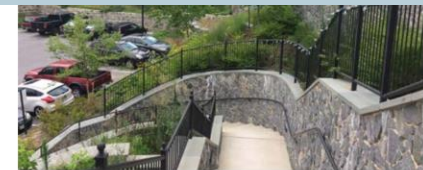
Figure 208: The Lot E Staircase Creates a Memorable Link Between the Courthouse Area and Main Street
