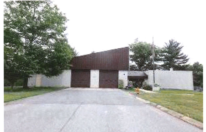
North Columbia Fire Station 03/25/2021
