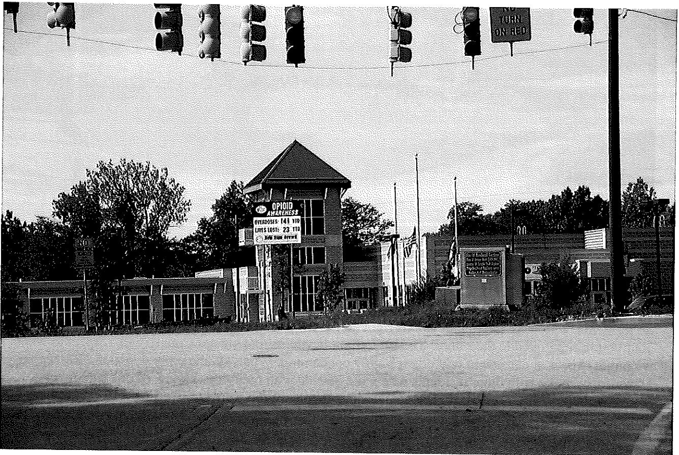
Exiting Lawyers Hill Road onto Montgomery Road. This is what Lawyers Hill Road residents view each time we leave our neighborhood.
