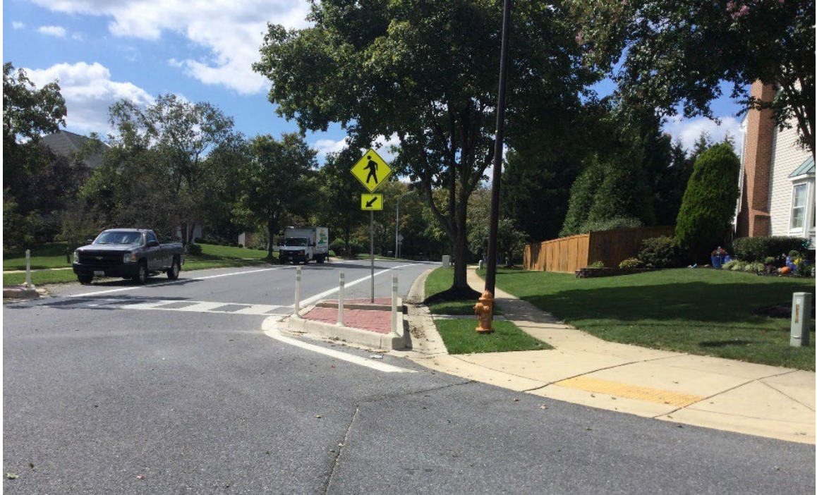
Figure 2-16. Intersection Curb Extension provided as a retrofit.
