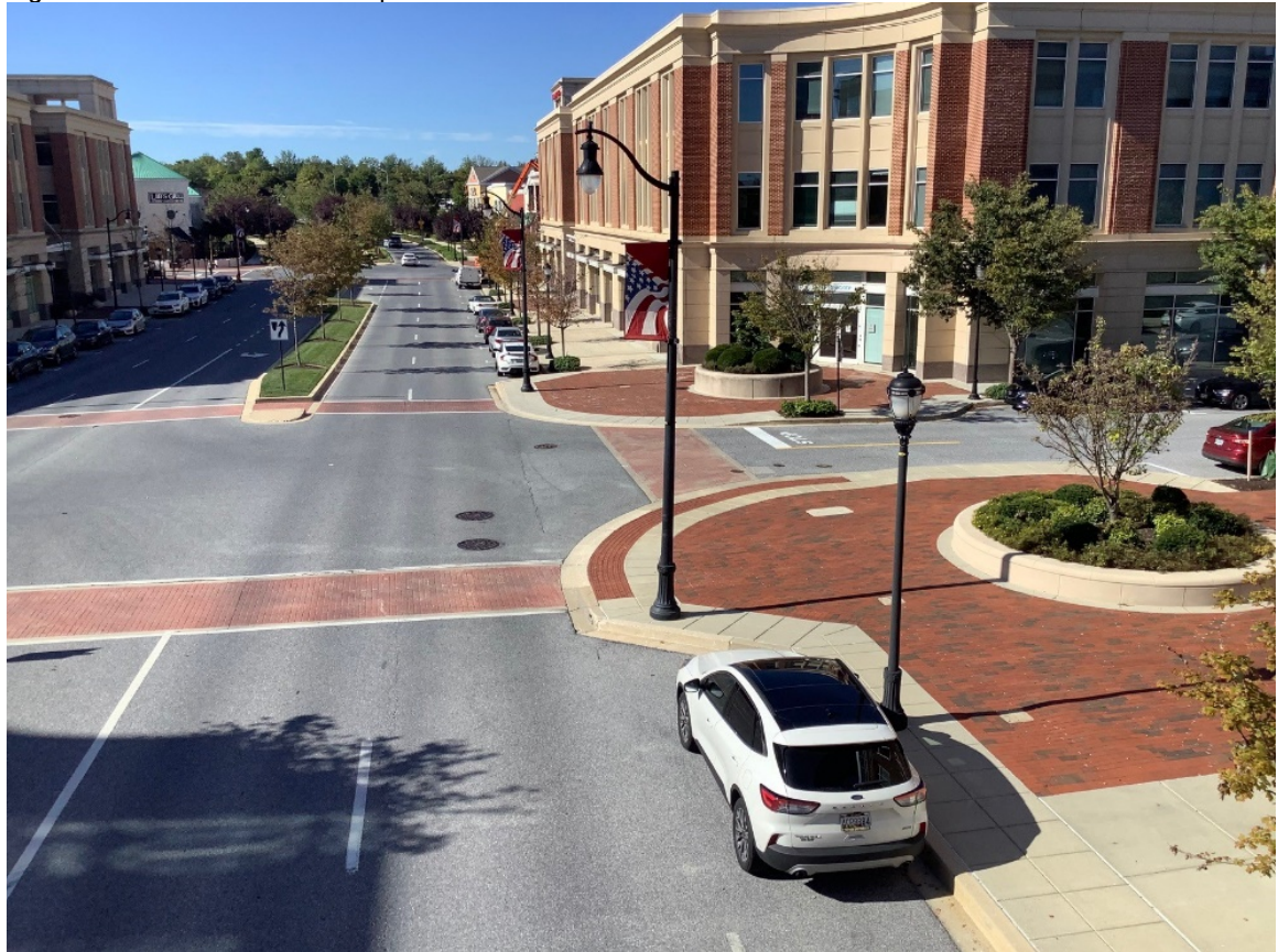
Figure 2-20. Mountable Truck Apron.
