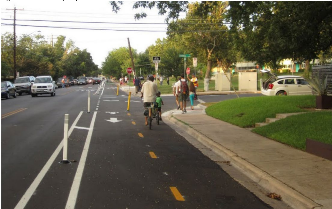
Figure 2-5. Two-Way Separated Bike Lane.
