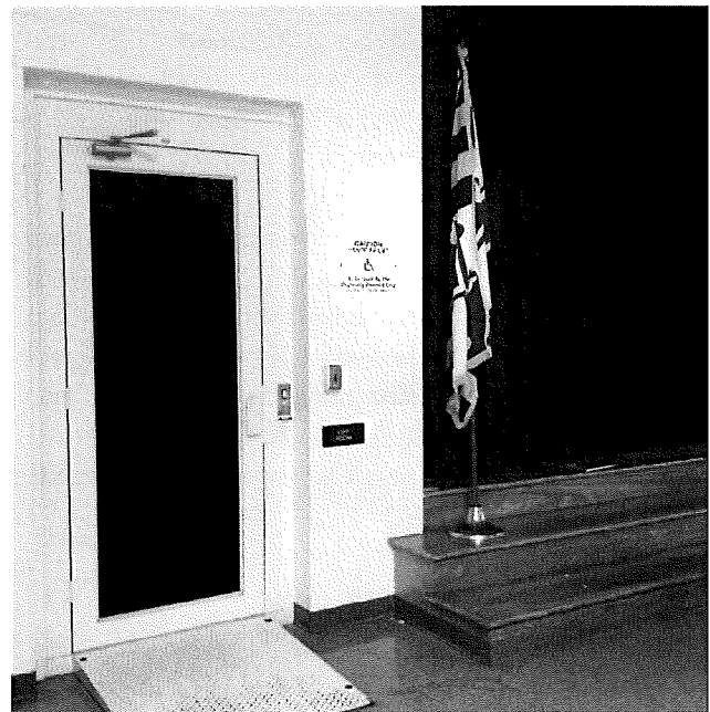
Lift room for access to the stage.
