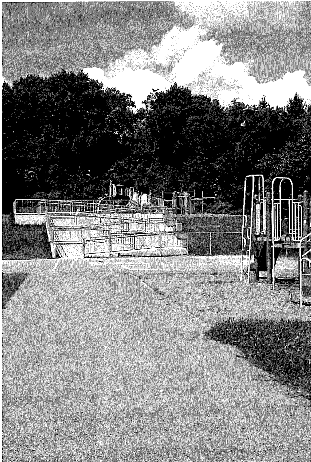
An accessibility ramp to access the upper level play area at Bryant Woods Elementary School.
