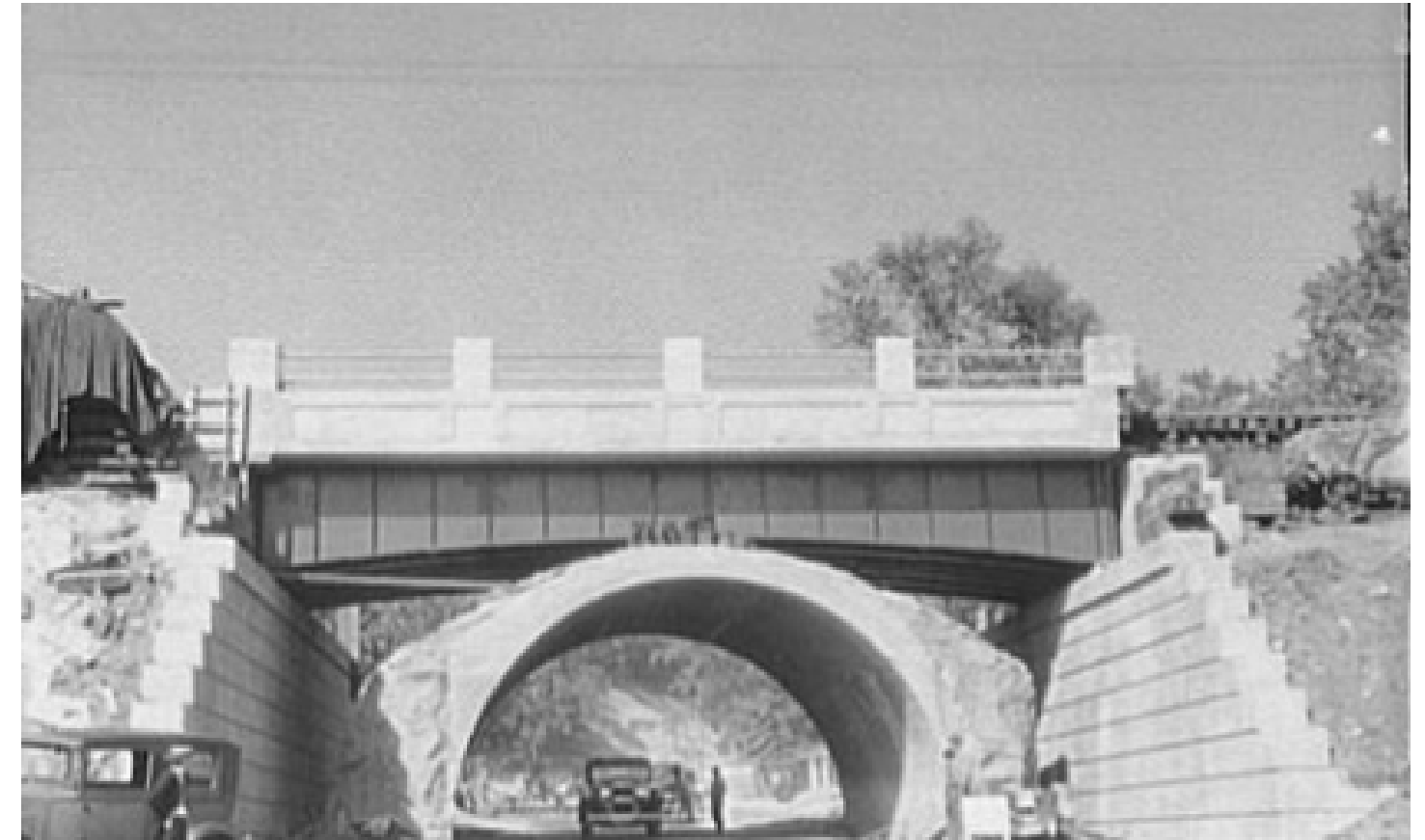
B&O Railroad bridge construction in Elkridge on Route 1, photo circa 1931.
