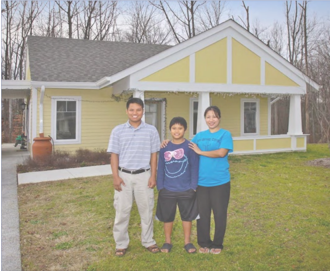
Image 6-1 is an example of a modest-sized home, approximately 1,300 square feet, in the Cottages at Greenwood, a permanently affordable housing development that consists of 10 single-family homes on approximately 3.5 acres. This development provides homeownership opportunities for moderate-income households. In 2011 and 2012, homes in the neighborhood sold for $252,400. In 2019, a home in the neighborhood sold for $265,274.
