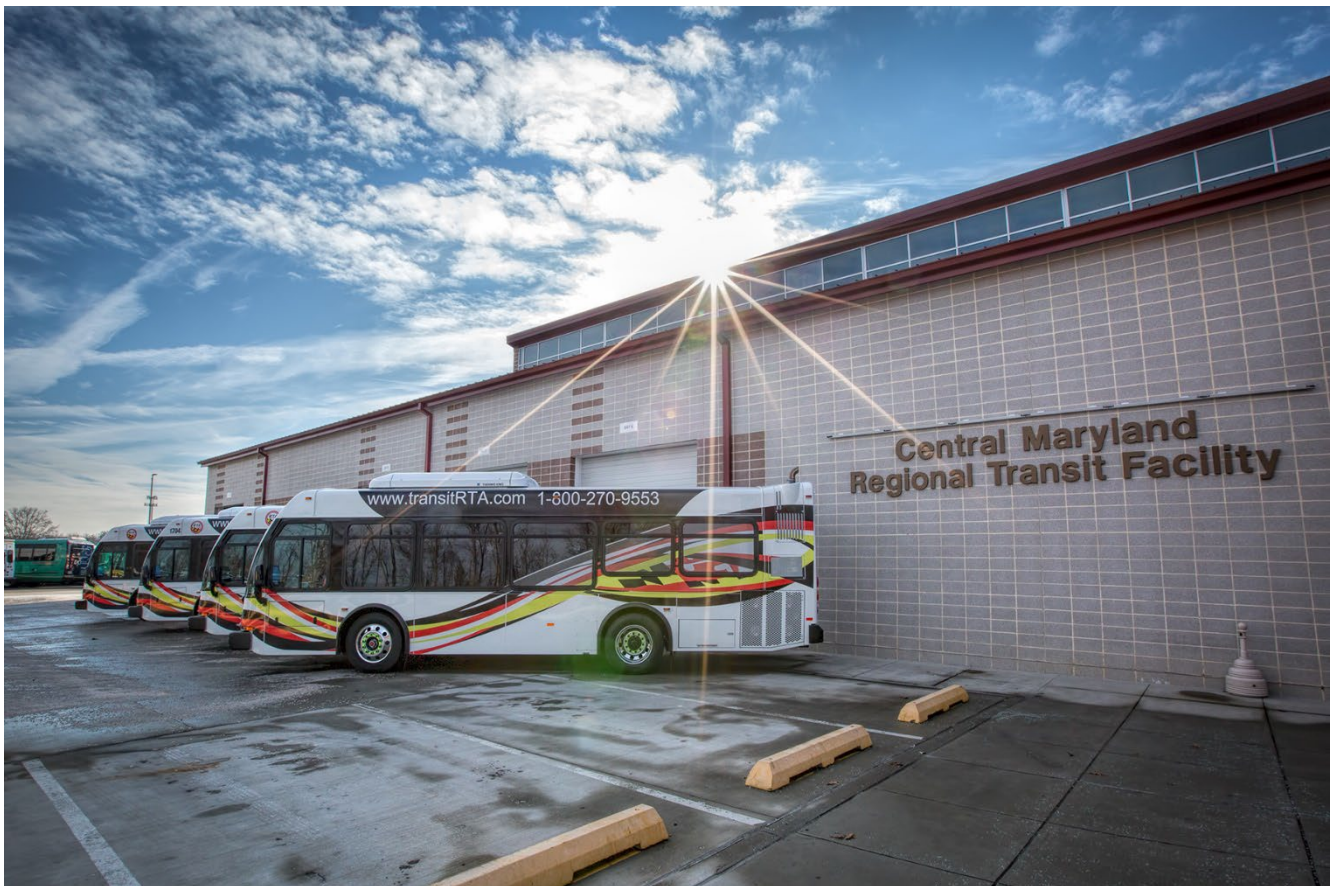
Figure 2-3: RTA Operations and Maintenance Facility (8800 Corridor Road)
