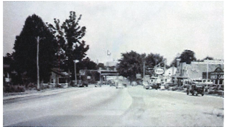
This portion of Route 1 was built in the 1920s to bypass Main Street Elkridge, photo circa 1940s.
