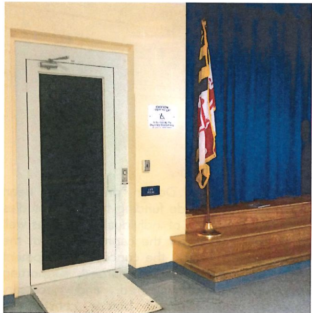
Lift room for access to the stage.
