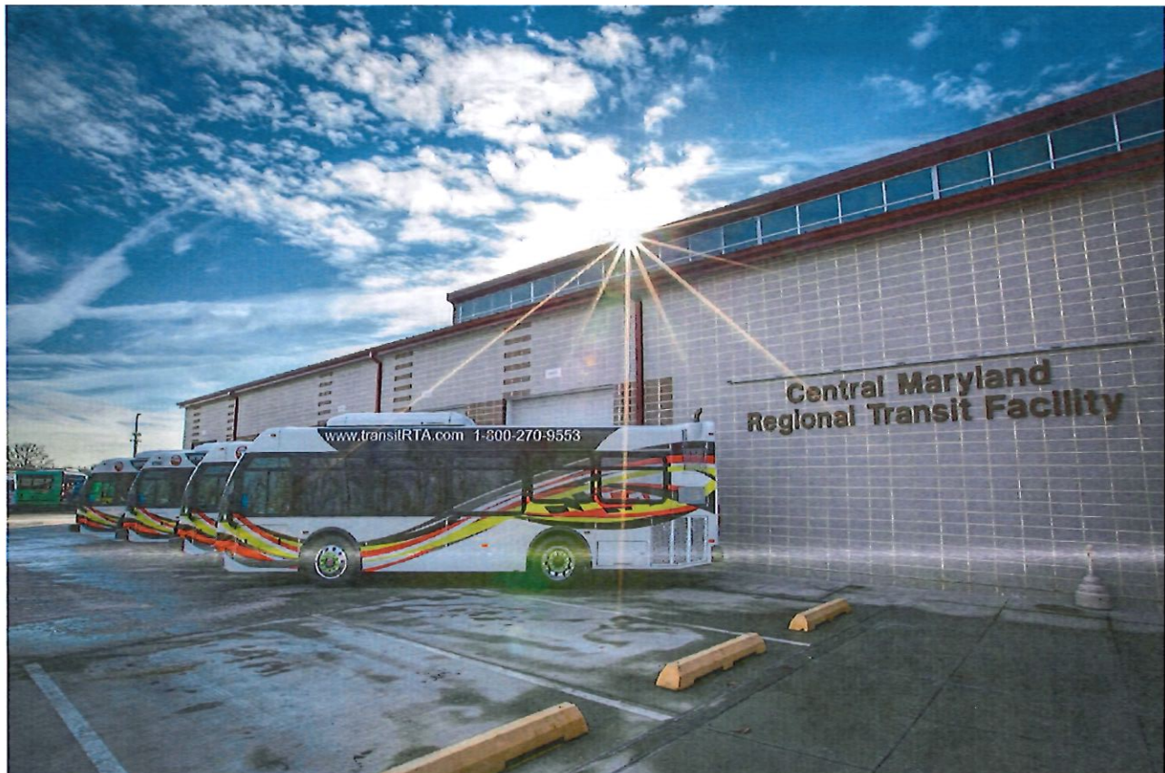
Figure 2-3: RTA Operations and Maintenance Facility (8800 Corridor Road)
