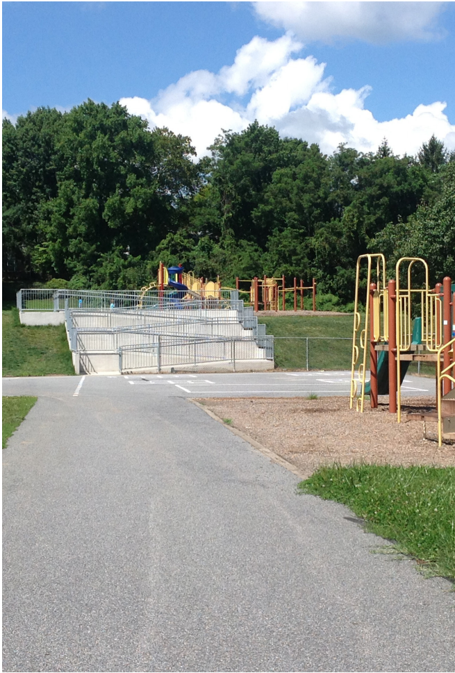
An accessibility ramp to access the upper level play area at Bryant Woods Elementary School.
