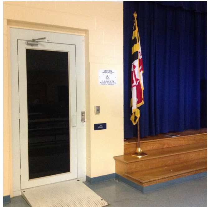
Lift room for access to the stage.
