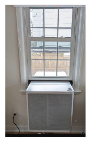
Looking to find solutions for New York Housing renters and residences in New York City's housing department ran an energy challenge. The winners were two manufacturers for cold-climate window heats pumps. These units use 120 volt outlets, don't block the window's view, can be installed in under 30 minutes. Costs \$3,800 each and heat and cool ~ 900 square feet. Midea and Gradient heat pumps.
