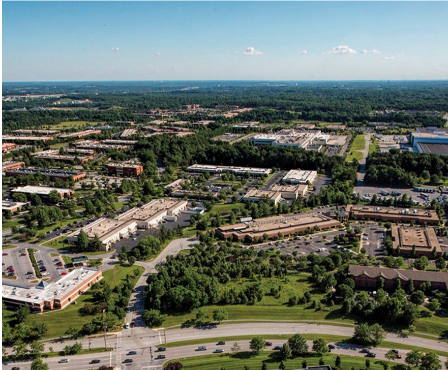
Figure 10: Aerial photo looking south from Columbia Gateway Drive
