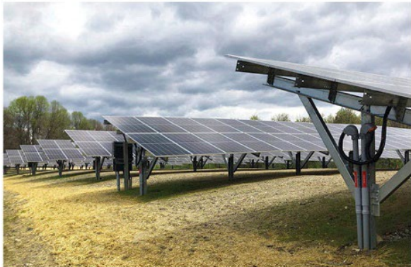
Howard County Circuit Courthouse: A LEED Gold-certified building with roof solar PVs (middle) and a solar field (bottom) designed to supply the facility with over 50 percent of its energy needs.
