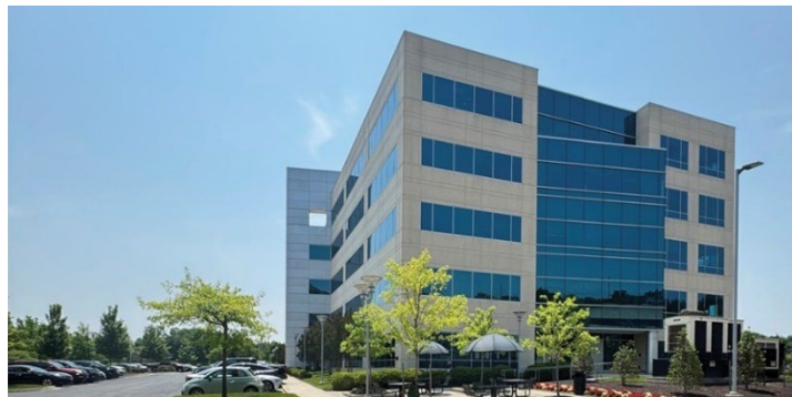
Figure 4: Existing office buildings in Gateway
