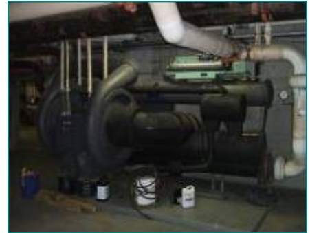
Existing Trane Centrifugal Chillers
