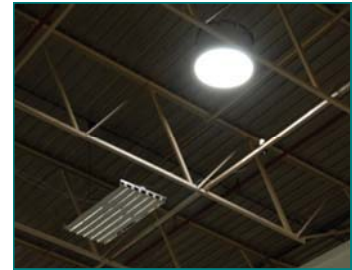
Light pipe installed
