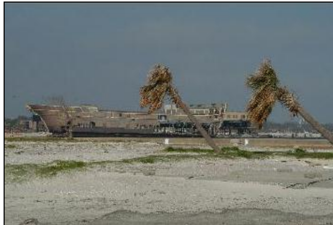
Figure A-8 Strong Wind Effects (Source: FEMA)
