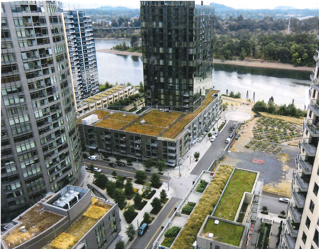
Figure 13. Ecorooftops at Portland's south waterfront neighborhood (Printed with permission ©2013 Environmental Services, City of Portland, OR)
