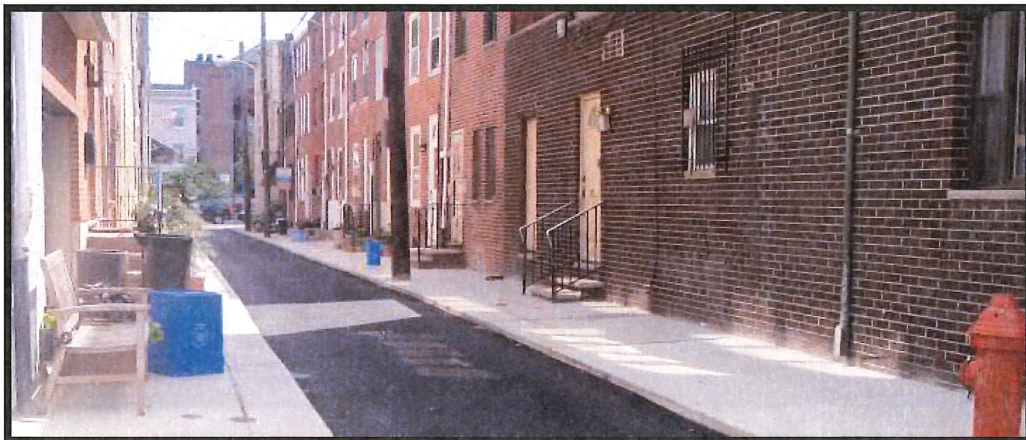
Figure 17: Porous pavement on Percy Street. (Photos courtesy of: Philadelphia Water Department)
