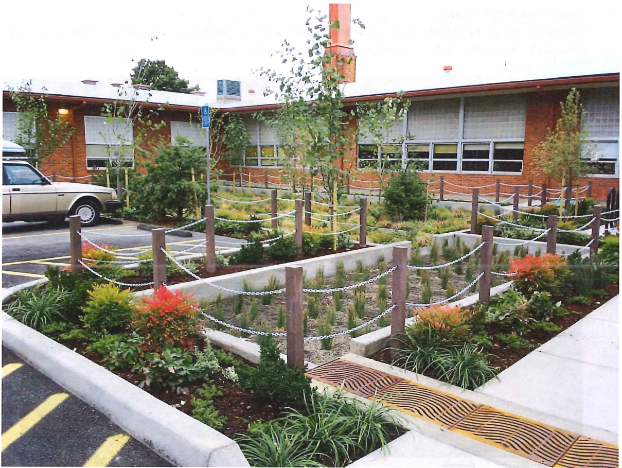
Figure 10. The Mt. Tabor Middle School rain garden in January 2007. The trench drain in the foreground delivers runoff from the asphalt play area (Printed with permission ©2013 Environmental Services, City of Portland, OR)
