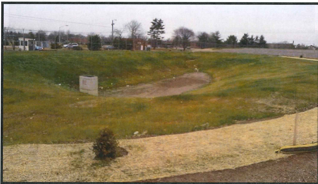
Figure 18: One of the vegetated detention basins built at Cardone Industries with the help of SMIP funds (Photo courtesy of: Philadelphia Water Department)
