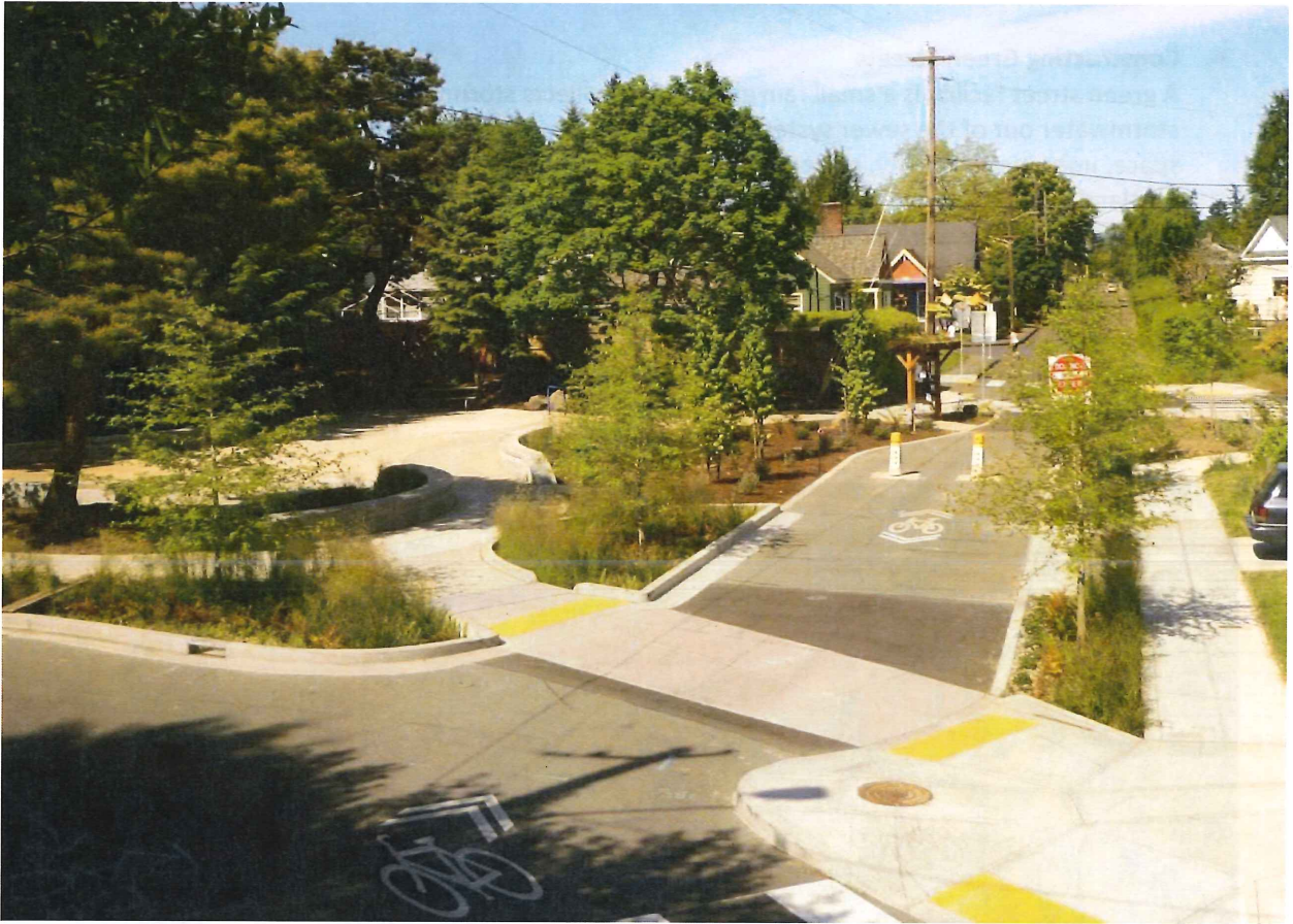
Figure 7. Part of the Holman Pocket Park and Green Street Bike Boulevard Project, two green streets in the ROW adjacent to the park accept runoff from the street (Printed with permission ©2013 Environmental Services, City of Portland, OR)
