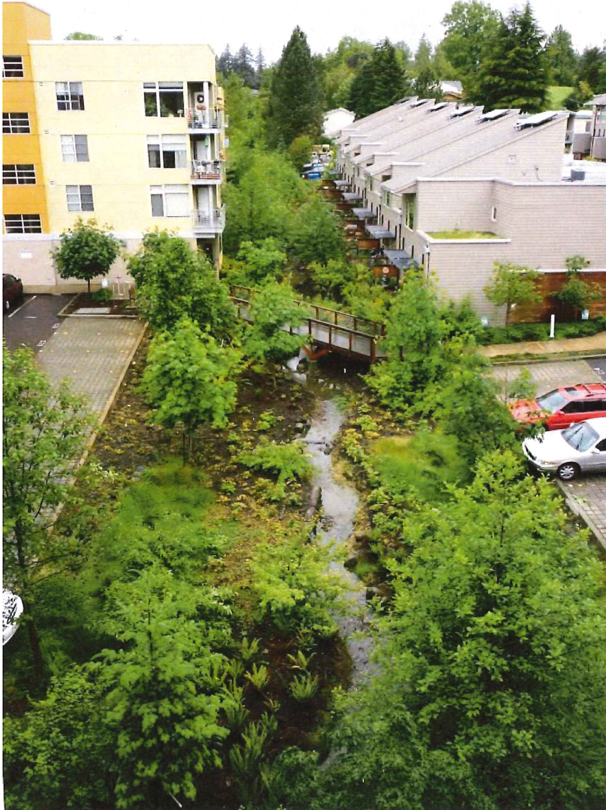
Figure 12. The Headwaters at Tryon Creek serves as a demonstration in sustainable stormwater management, green development practices, wildlife habitat restoration and water conservation. The daylighted tributary stream of Tryon Creek originally ran through a pipe under the site is approximately 450 linear feet, connects an upstream, forested wetland to a downstream rain garden, is planted with native trees, shrubs, and grasses that restore lost riparian and wetland habitat, and has a 5 foot (1.5 meter) deep gravel lens below the stream bed that helps direct flow below the surface for groundwater recharge (Printed with permission ©2013 Environmental Services, City of Portland, OR)
