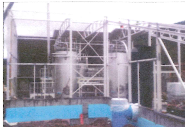
Figure 5: THP at Lindum under construction
