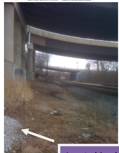
Locate bicycle path near bridge supports of MD 32 overpass
